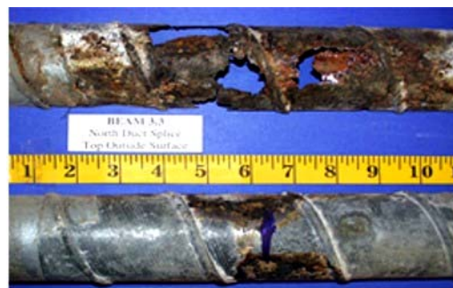
Figure 5.32: Specimen 3.3 – North Duct Splice
