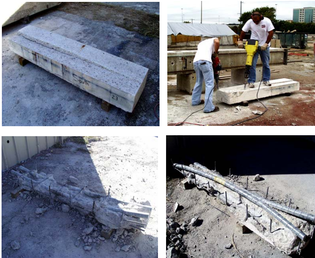
Figure 5.4: Concrete Removal and Reinforcement Exposure
