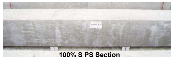
Figure 4.1: Typical Crack Patterns for Each Section Type 2
